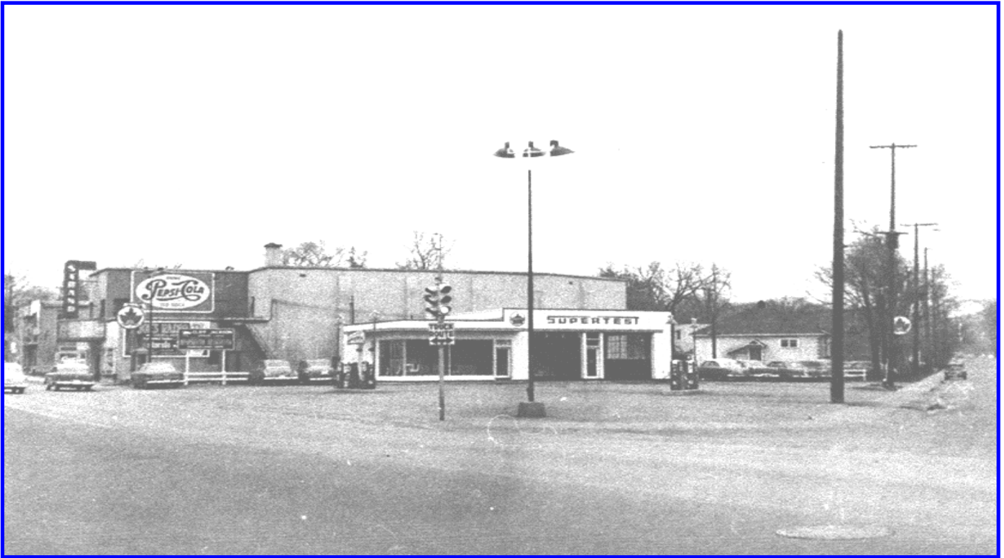
1305 Bank Street at Riverdale Avenue circa mid 1950s
