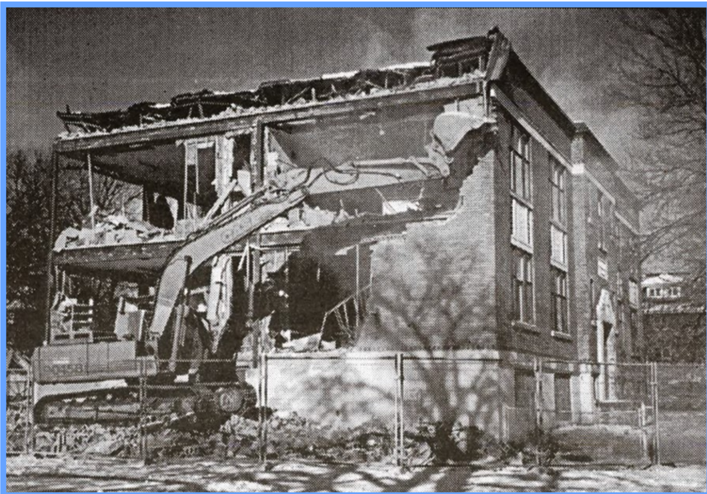
Demolition of St. Margaret Mary Catholic School in December 2004
