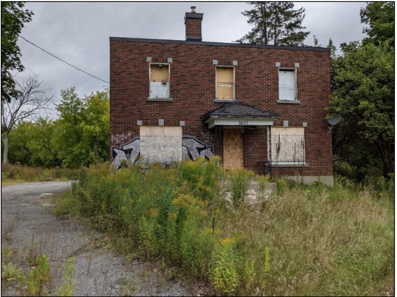
The Lefebvre House before demolition, 3637 Bank Street, September 2, 2021.
